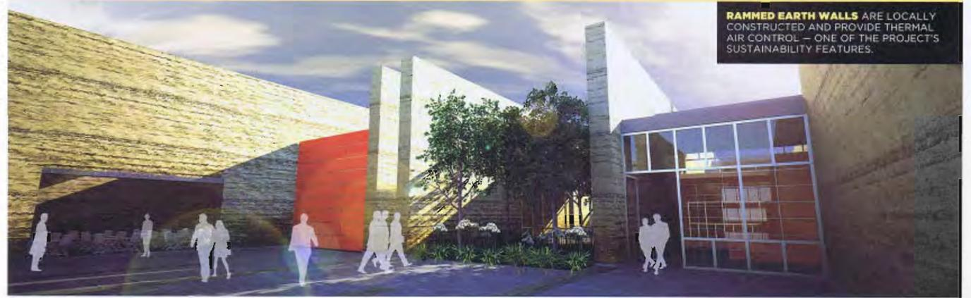
**RAMMED EARTH WALLS** ARE LOCALLY CONSTRUCTED AND PROVIDE THERMAL AIR CONTROL – ONE OF THE PROJECT'S SUSTAINABILITY FEATURES.
